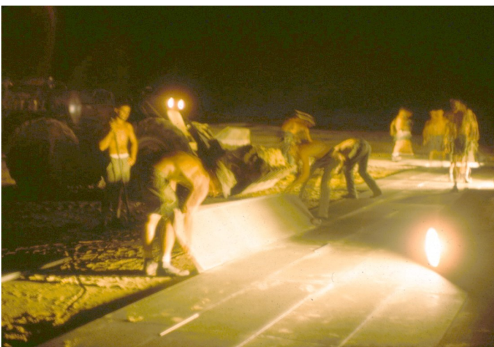
Seabees building an expeditionary airfield. All photos: Fred Quarnstrom
