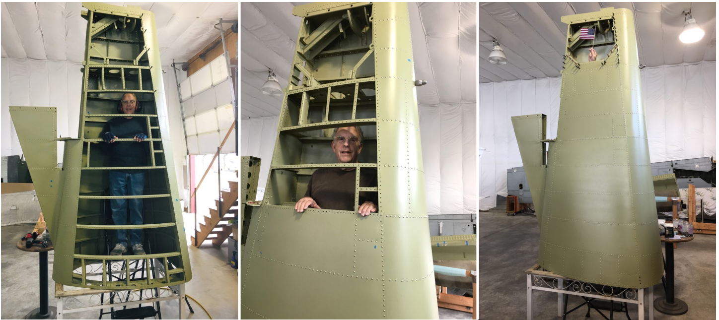
Jack slowly riveted himself into a corner while reskinning the empennage. Help! Photos: Jack LaBounty
