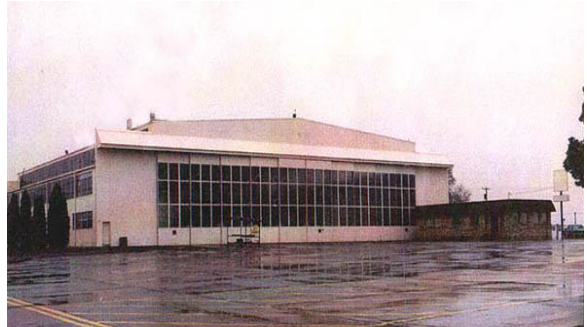
Bldg #113 at Pendleton is the hangar that the famed Doolittle Raiders operated from.
